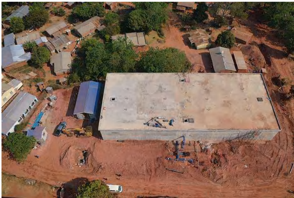
Progress of construction at St Maria Goretti Reservoir, 5,000m 3
