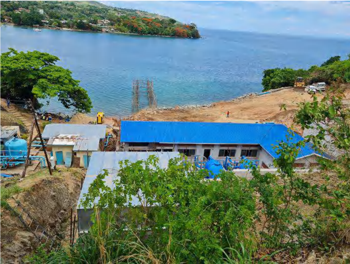
Progress of Construction at Water Treatment Plant
