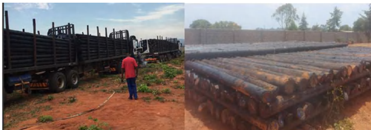
Figure 39: Some of the Malawi Electricity Access Project Materials
