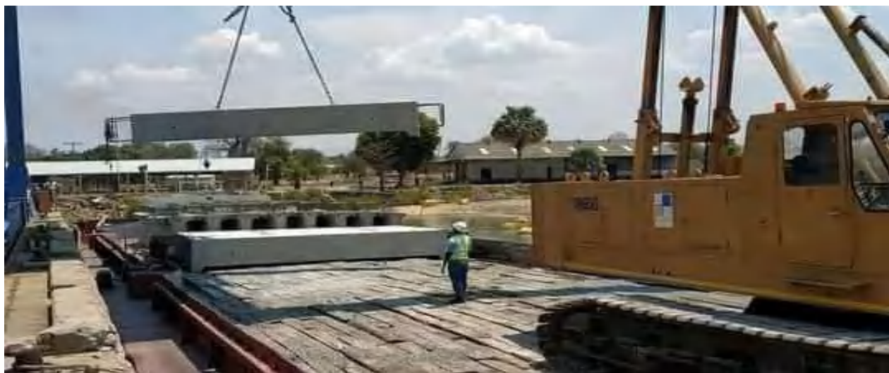
Figure 32: construction of Likoma jetty
