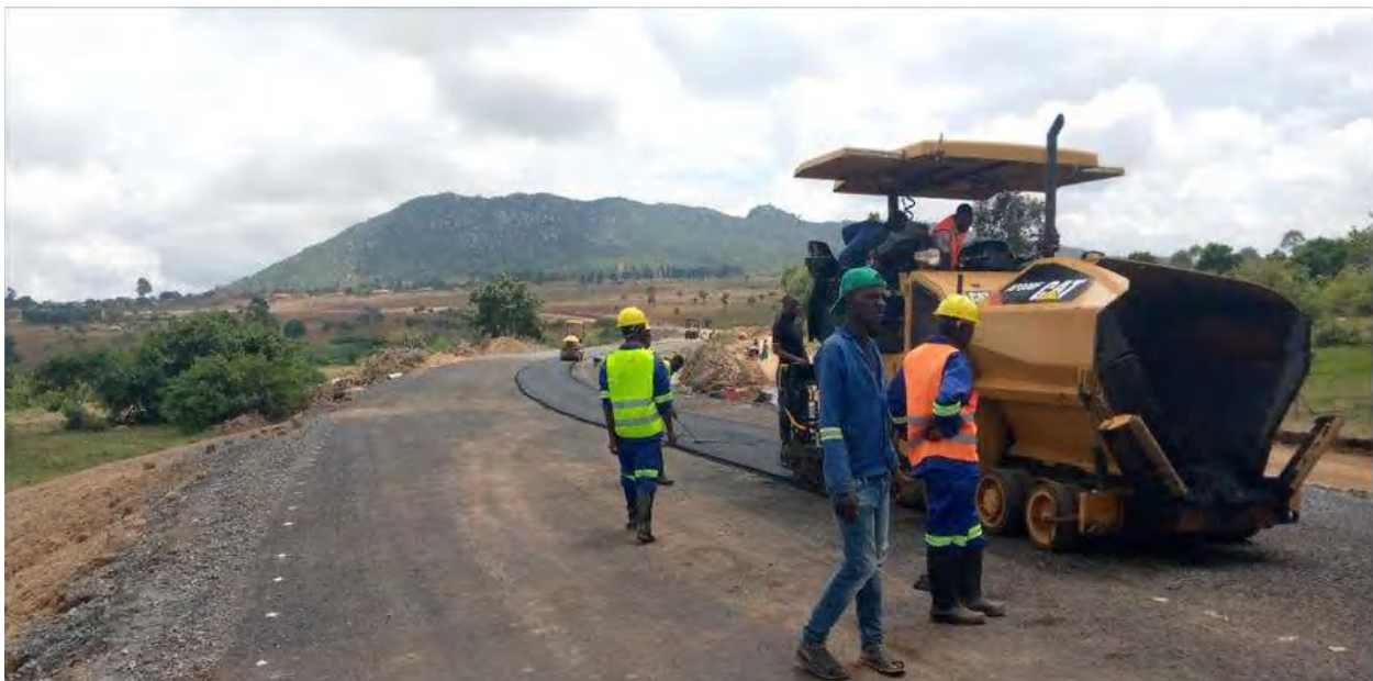
Figure 53: Works on One of the Sections of the Road
