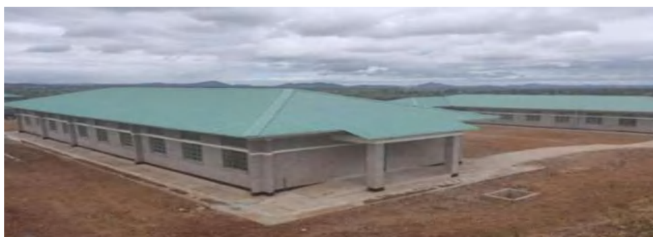
Figure 45: Constructed Blocks Under the Project
