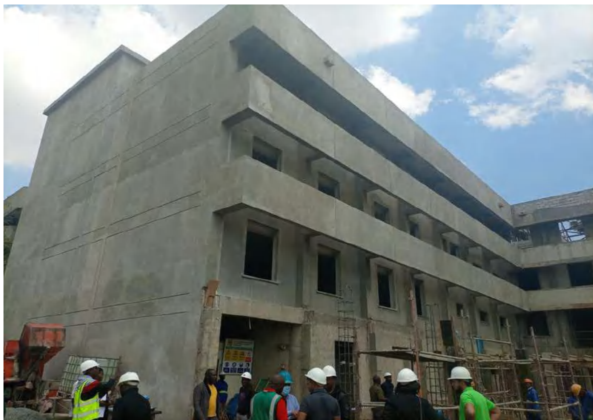
Figure 37: Construction of the new Blantyre police station
