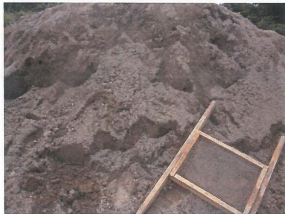
Sieve sand to remove plant roots
